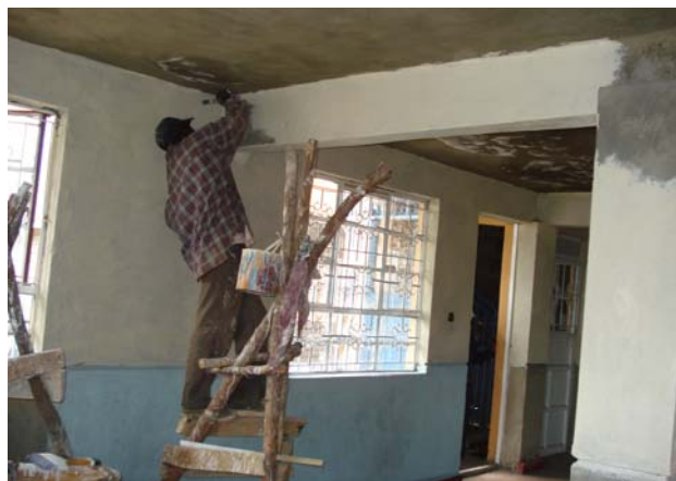
Painting on progress
